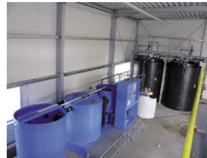
ADF-flotation with chamber filter-press for surface dewatering at storage areas or transshipment spaces of discarded metal with adherence of emulsion.
