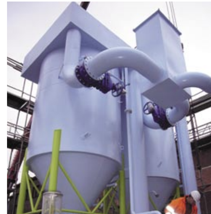
Galaxie-Tower for process- and circulation water treatment.
