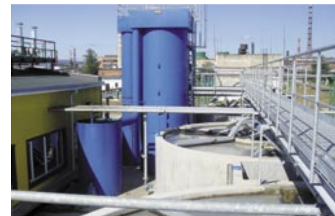
Galaxie-Tower for process- and circulation water treatment.
